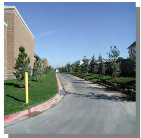
Secondary Access Road
