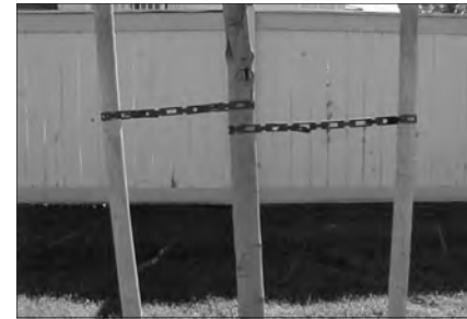
Figure 14 – Good staking
