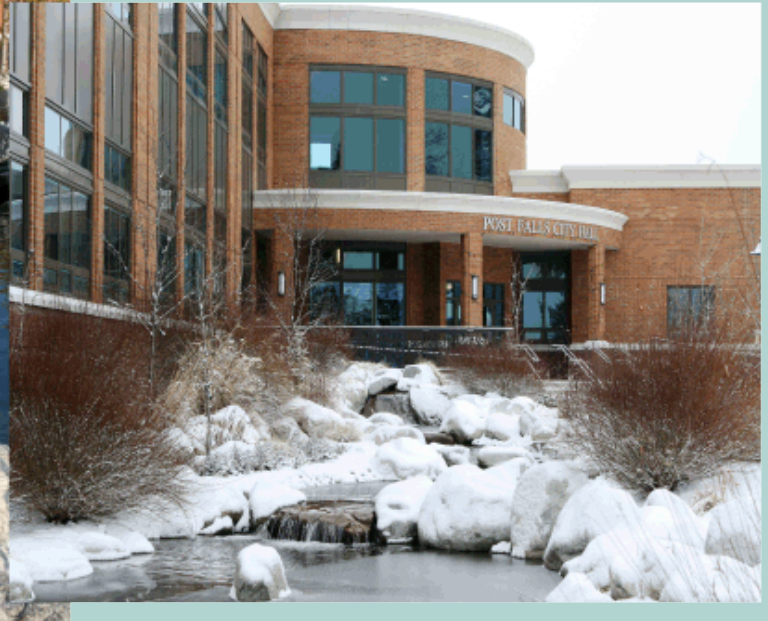
Above: Post Falls City Hall Plaza in Summer and Winter
